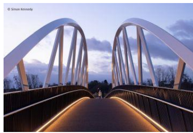
Figure 9. Hams Way Pedestrian bridge, Source: (Hams Way, 2021).
