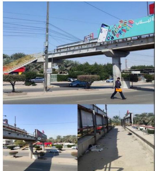
Figure 14. Al Ghadeer Maysaloon pedestrian bridge (Source: Authors).
