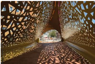
Figure 8. Copr Bay Pedestrian Bridge, Swansea, Source: (Copr Bay, 2021).
