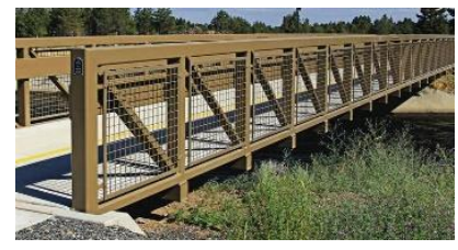
Underhung- bridge design
