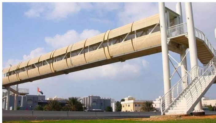
Figure 6. A pedestrian bridge in Abu Dhabi city, Source: (Youmone, 2022).
