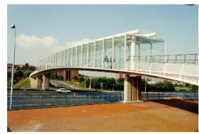
Figure 10. Enclosure at Oldham Way Pedestrian bridge, Source: (Oldham, 2019).
