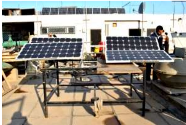
Figure (3) show the panels in roof building
