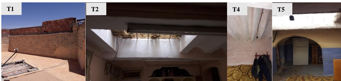
Figure 10. Comparison of materials used after renovation or modification: on the left, T1 and T2 with industrialized materials (concrete block, brick, cement, steel beam); on the right, T4 and T5 preserving traditional materials (stone wall, lime, palm beam). Source: (Photos by Authors).
