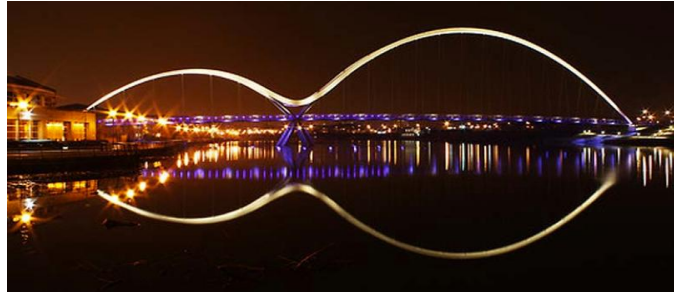
Figure 6. Infinity Bridge in Stockton-on-Tees, composed of two asymmetrical arches. Its name derives from the water reflection that creates an infinity symbol [22].
