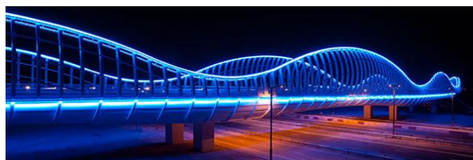
Figure 9. Dubai Meydan Bridge (Rope lighting) [26].
