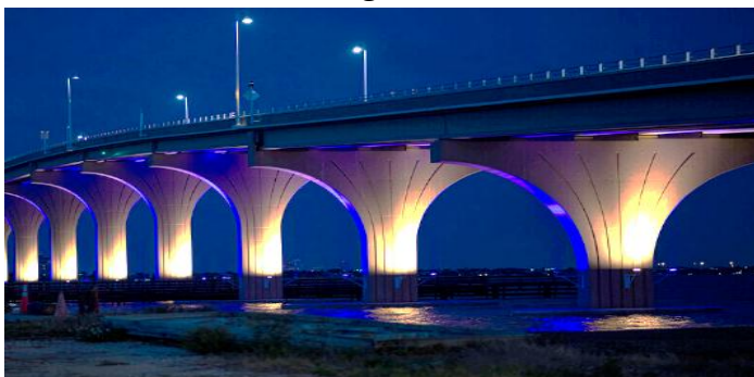
Figure 11. Pinellas Bayway Bridge (up lighting) [11]
