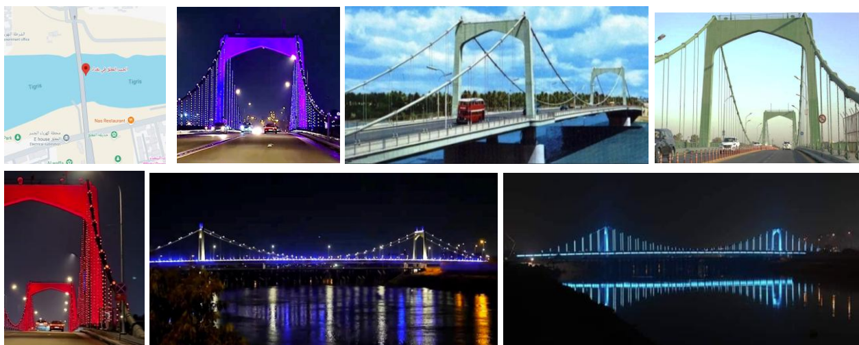
Figure 13. Artificial Lighting Techniques of 14th of July Bridge.
