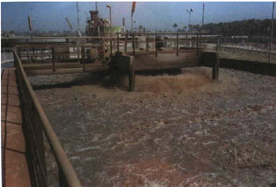
Fig. 4, High Mixing Rate With the New Drive Motors of 1500 r.p.m. 55 Kw. (after Brochier (4) )
