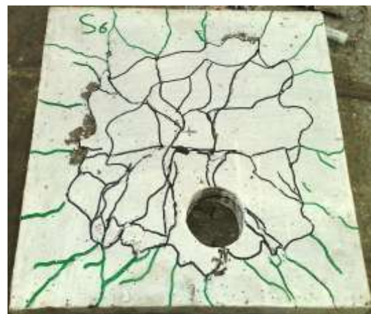
Fig.(20) Crack Pattern at Failure for Specimen S6.
