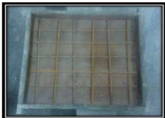
a. Steel Bars & Mould
