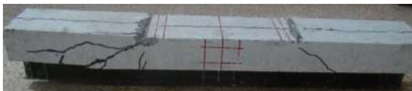
Figure (7) Failure Shape of Tested Beams Sample
